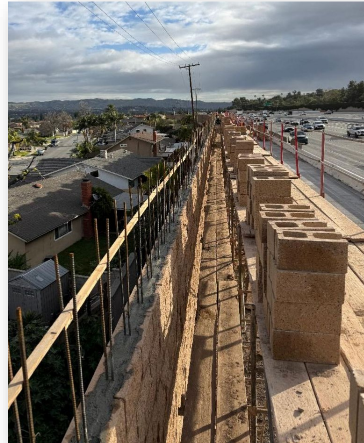
Preparation for placing blocks that form the top of the sound wall along the westbound SR-91 on-ramp
