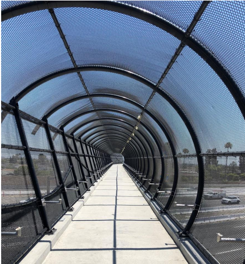
Heil Avenue (pedestrian) bridge construction
