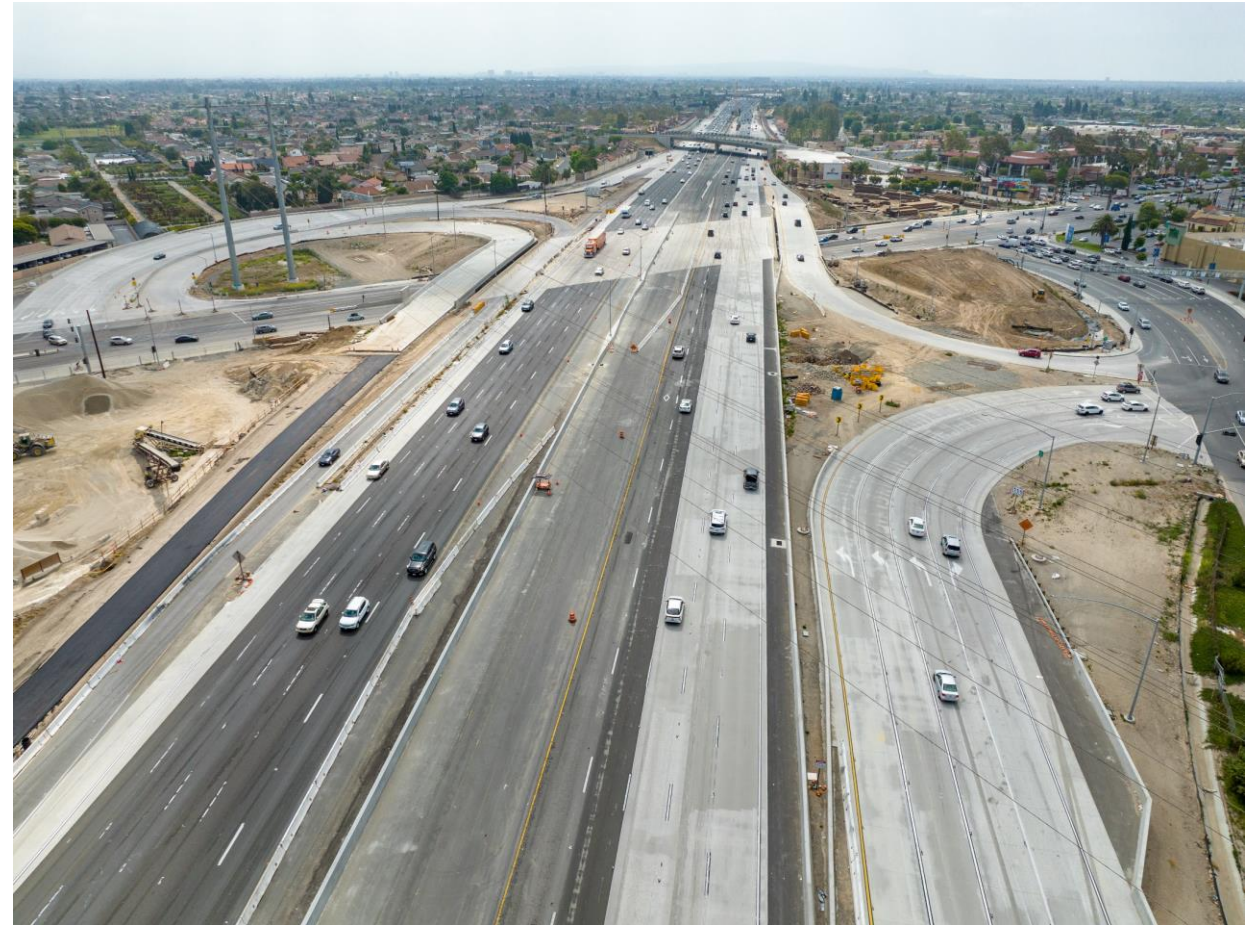
Beach Boulevard construction
