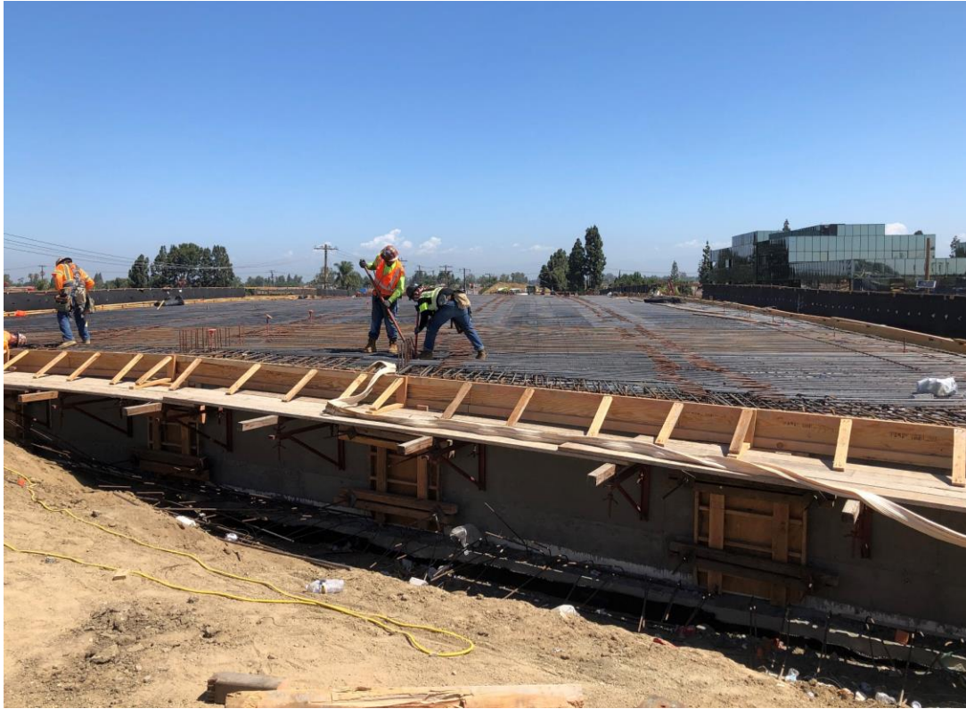
Ward Street bridge construction
