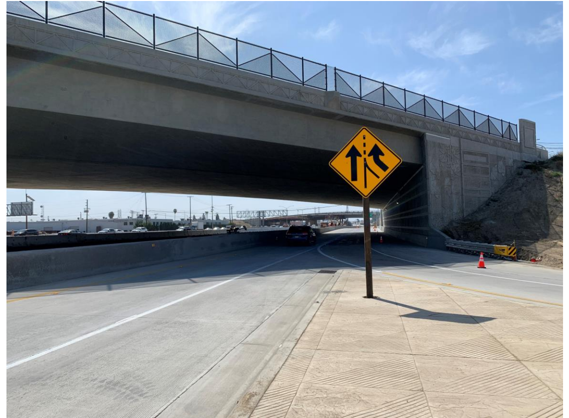
Goldenwest Street bridge construction
