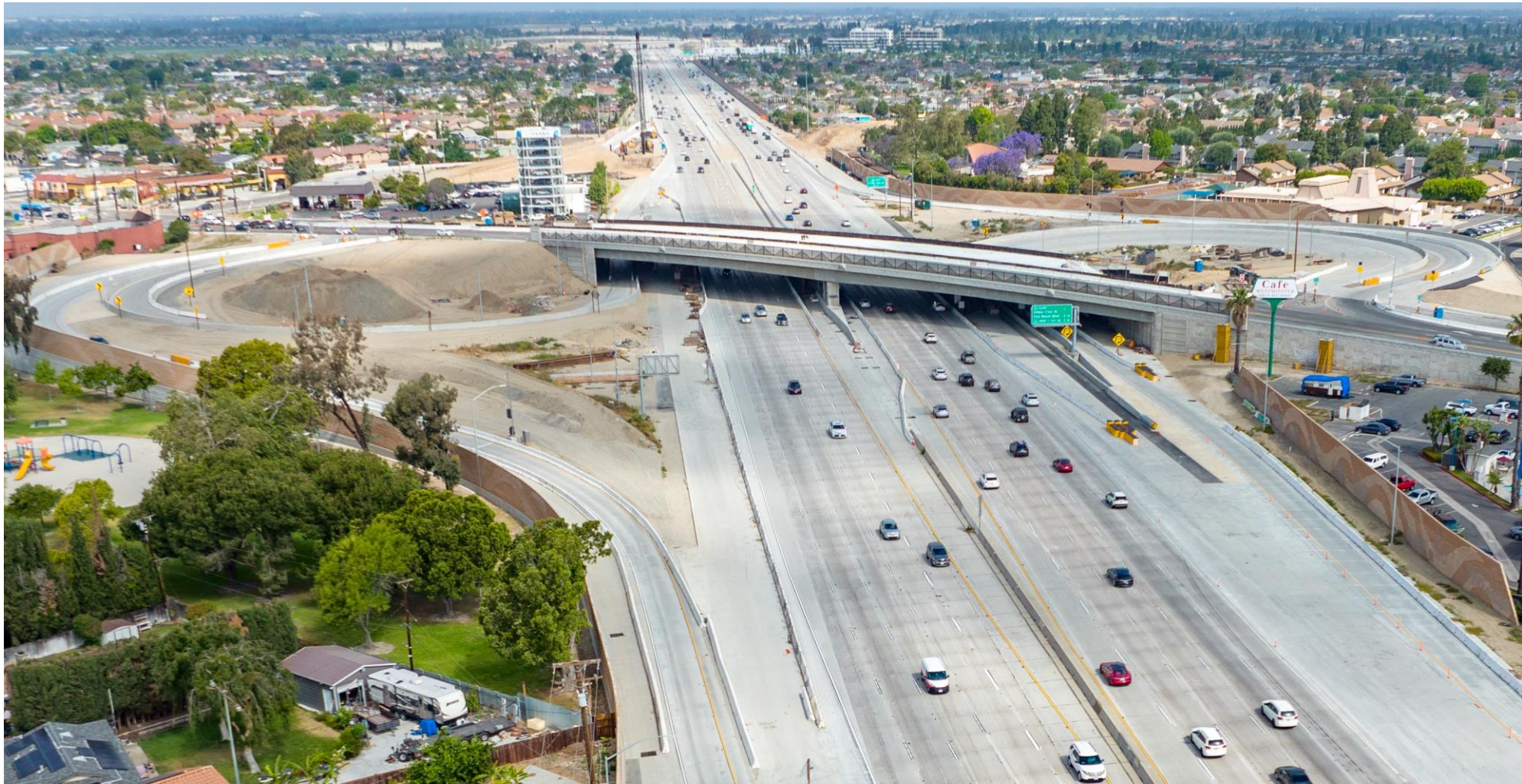
Westminster Boulevard bridge construction
