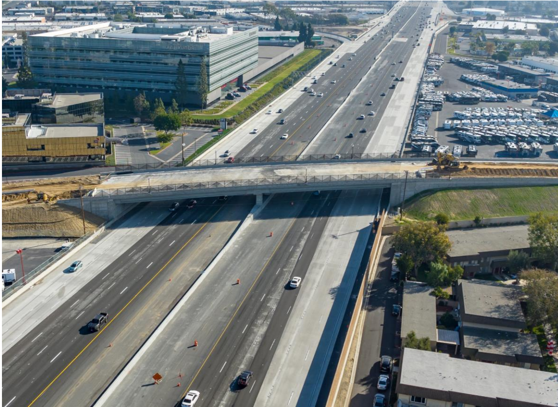
Ward Street bridge construction
