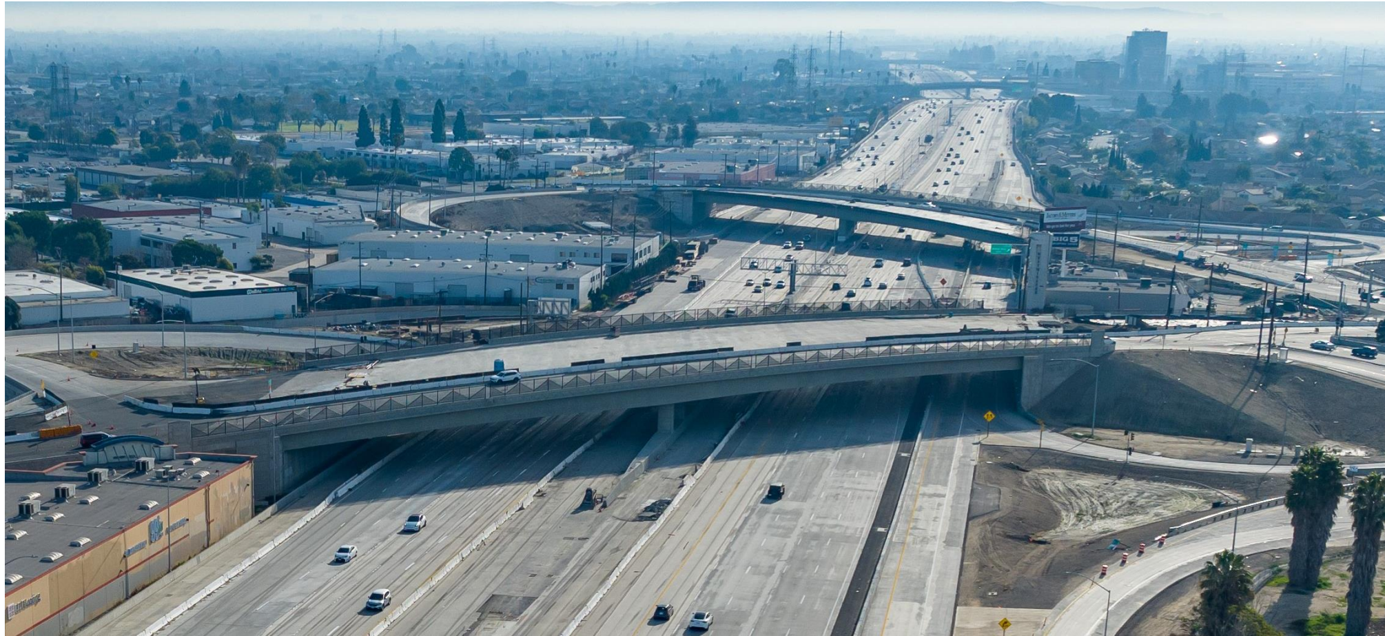
Bolsa Avenue and Goldenwest Street bridge construction
