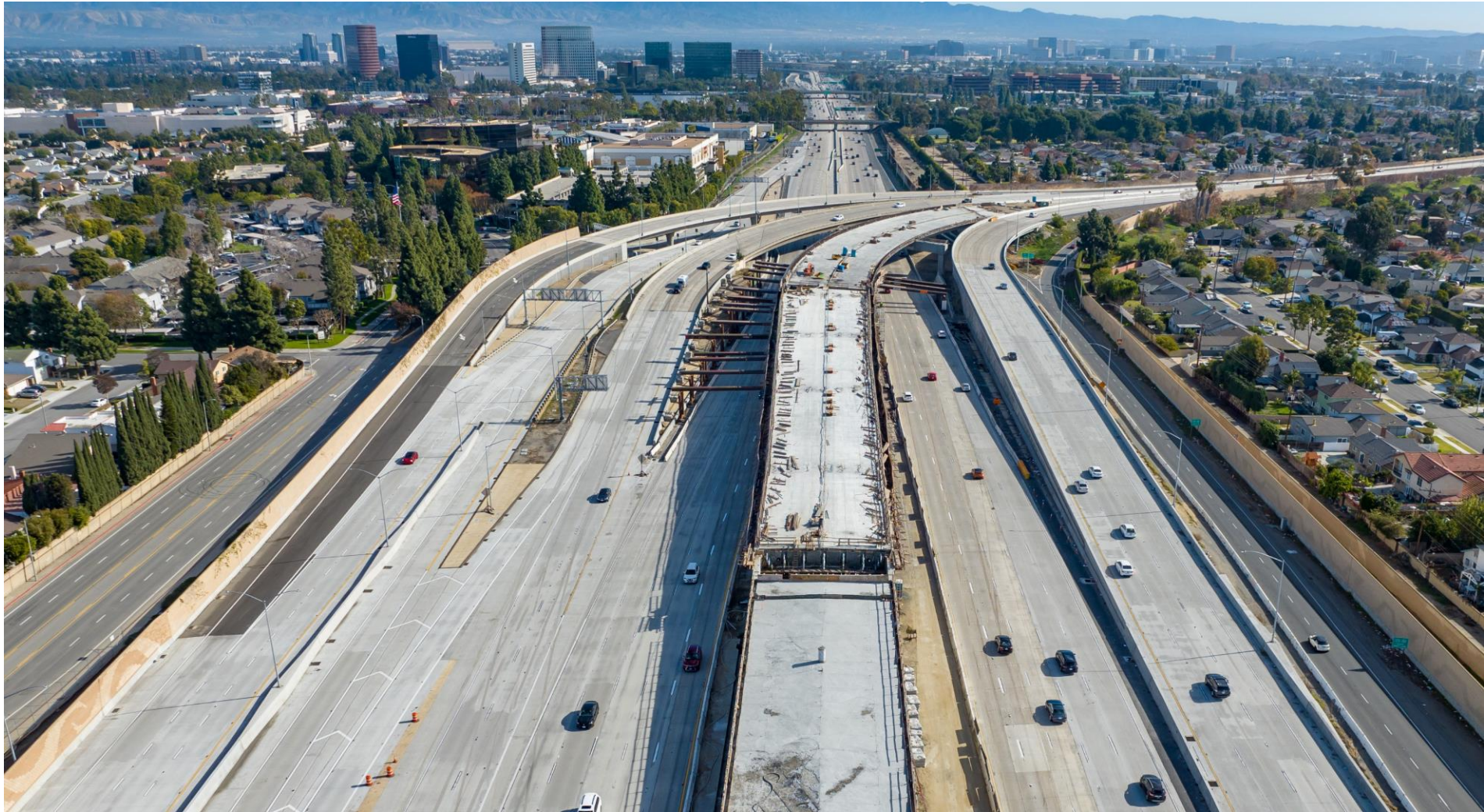
I-405/State Route 73 (SR-73) median connector bridge construction
