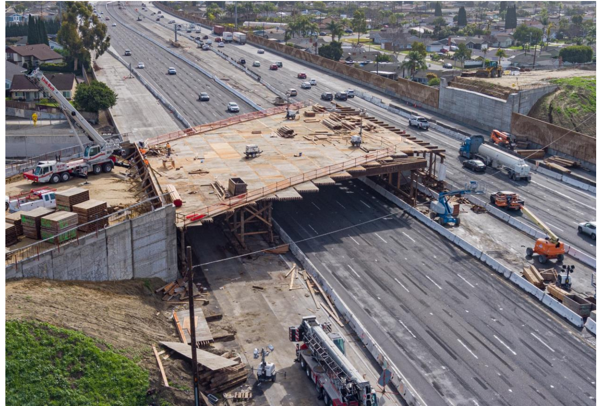
Newland Street bridge construction
