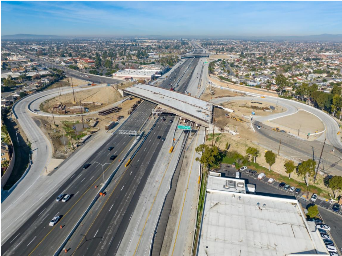
Warner Avenue bridge construction
